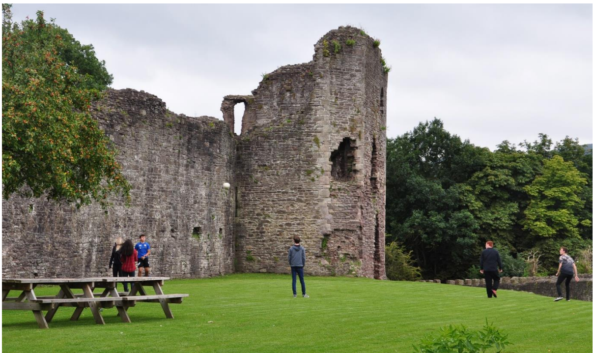
Lawn in front of Curtain Wall - View right immediately after entering castle grounds
